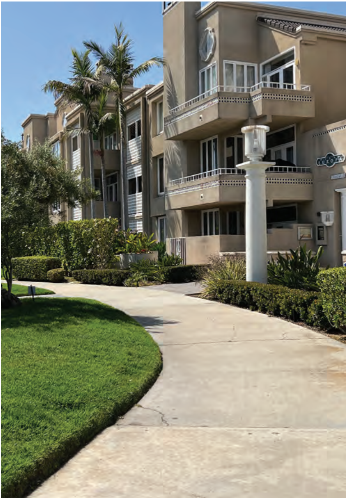
Accessible, interconnected pedestrian routes improve walkability.
