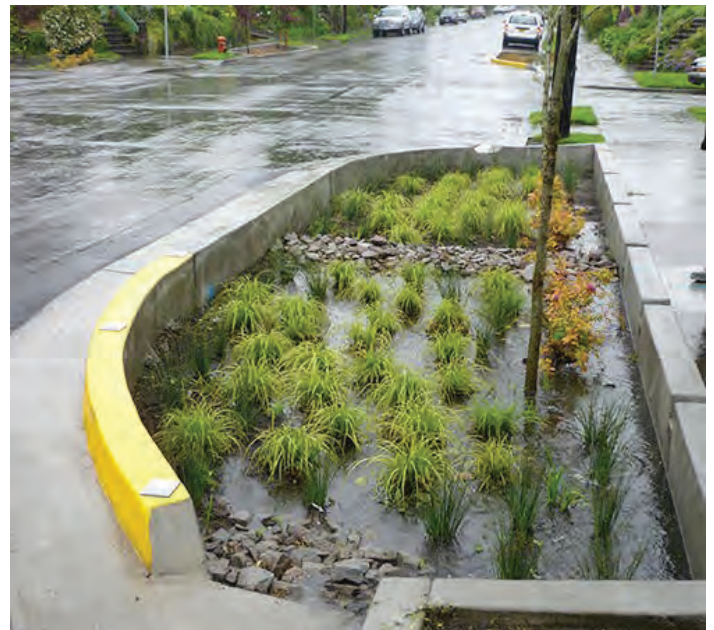
Green infrastructure like stormwater detention basins help mitigate stormwater runoff and flooding.
