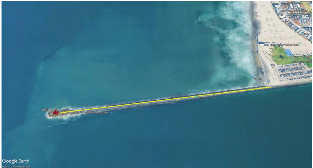
Pictures 6 & 7 - Overview of Jetty Walk Extraction (yellow)
